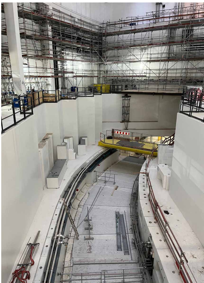
Super-FRS target area under construction at FAIR.
